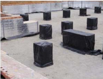
Sealed Crawl Space
